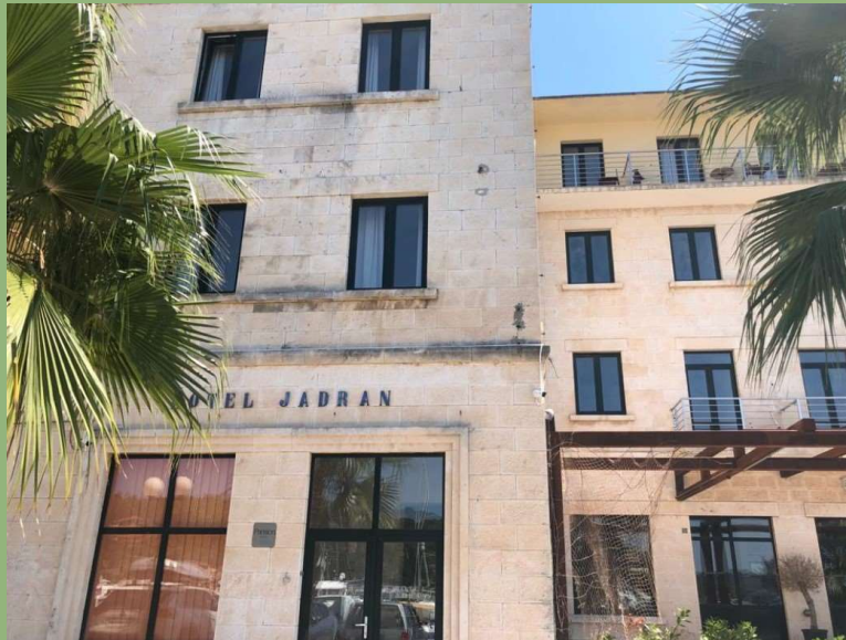
Ground Floor view
